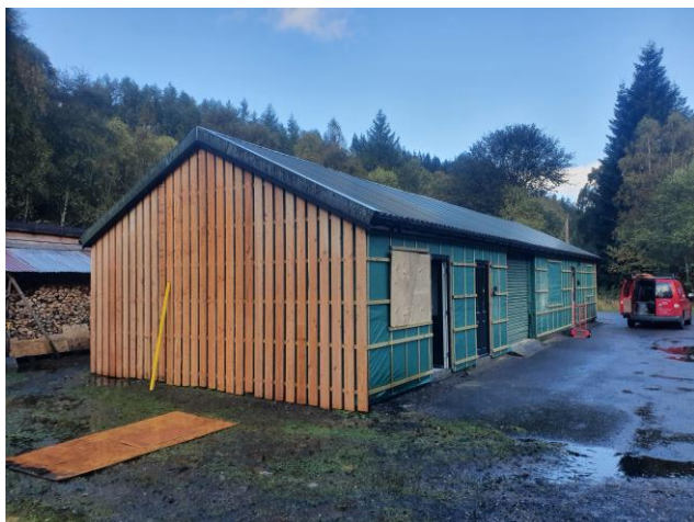
Larch cladding started going up in early October
