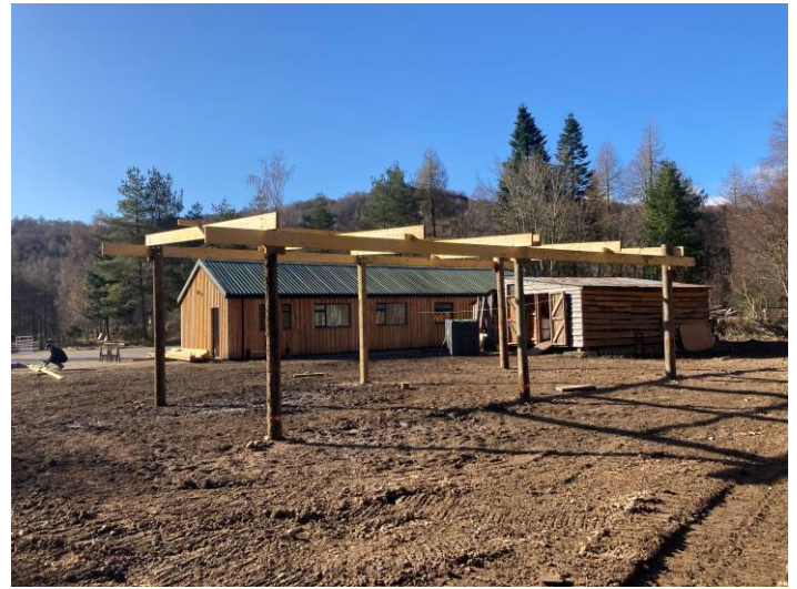
The shed frame goes up in early April
