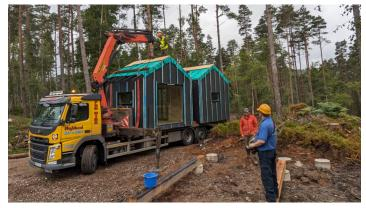
The next stage for the cabins is to put the cladding on; this is the larch that we've milled from out own timber in the community woodland, and it'll start going up in the next couple of weeks. North Woods Construction will be back to install the stoves and other internal works over the winter. In the meantime, we're about to start work on the amenity building (showers, kitchen and lounge) very soon.
