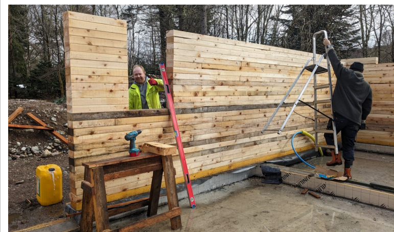
The amenity building under construction.
